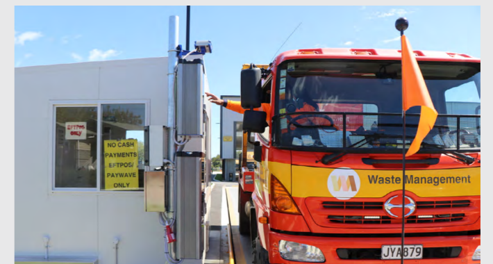
The unmanned weighbridge utilises number plate recognition technology and an automated kiosk for payment.
